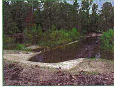
CANAL 2 SPILLWAY COMPLETED 9/2005
