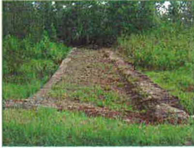
CANAL 2 AT REYNOLDS
